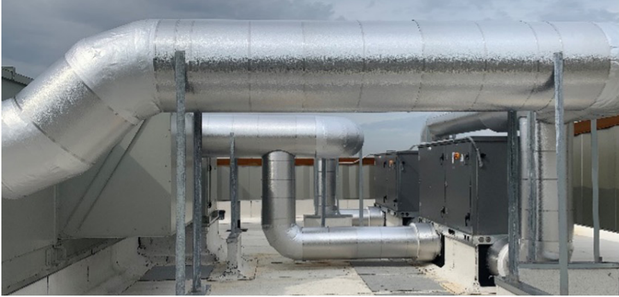
Figure 2: HLR Module installed on the Solis-Cohen Elementary School roof
